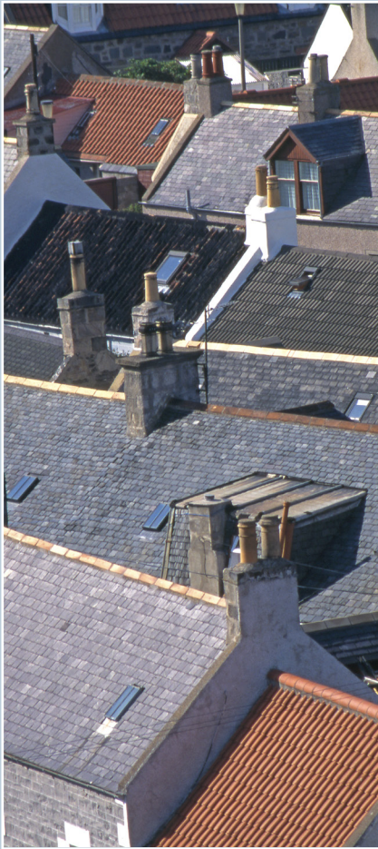
The Seatown at Cullen, Moray, showing a wide range of slated and pantiled roofs. The Scots slate here is darker and smaller than the more regular blue Welsh slate. Pantiles were commonly used in Eastern Scotland where cheaper and well-ventilated roofs were needed, but slate was preferred on most houses.
