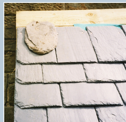
Sample panel prepared to ensure appropriate grading and random widths in the laying of new slate, with a fire-damaged Perthshire slate from Morgan Academy, Dundee.
