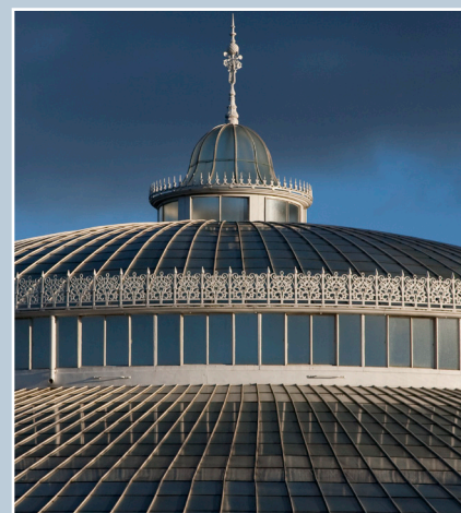
Glazed roof at the Botanic Gardens, Glasgow City. © N. Haynes.
